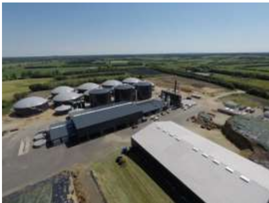
Figure 1: Biogas plant – Photo: Lundsby - Vinkel Bioenergi
